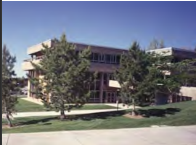
Bennion Administration Building
