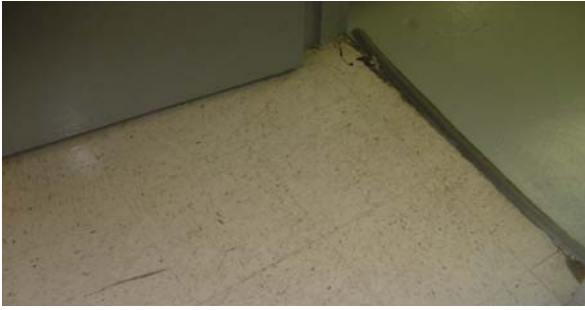
Photograph 1- M001 12" Floor Tile, White w/Gray Streaks, No Mastic Hallway 106A, Room 106
