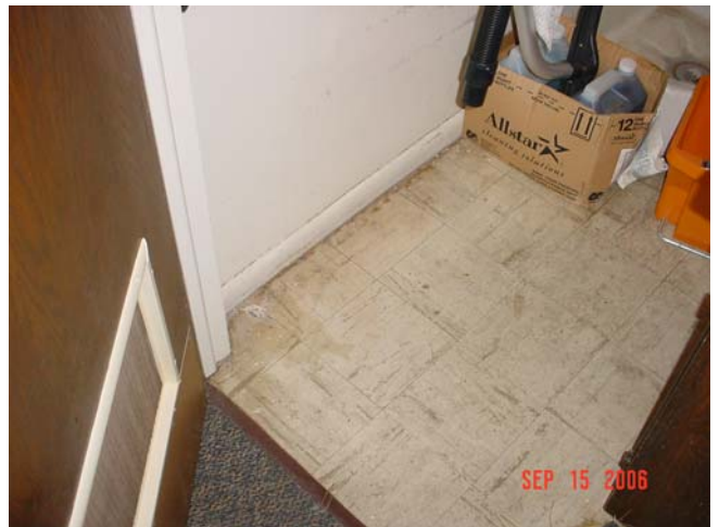
Photograph 6-SUU FACILTITES/AUTO Room 107 custodial closet, M002, 9" floor tile, exposed, ACM.
