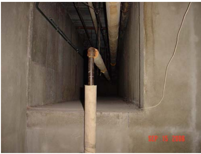
Photograph 1-SUU FACILTITES/AUTO Room 001, TSI pipe lagging (fiberglass, NON-ACM).
