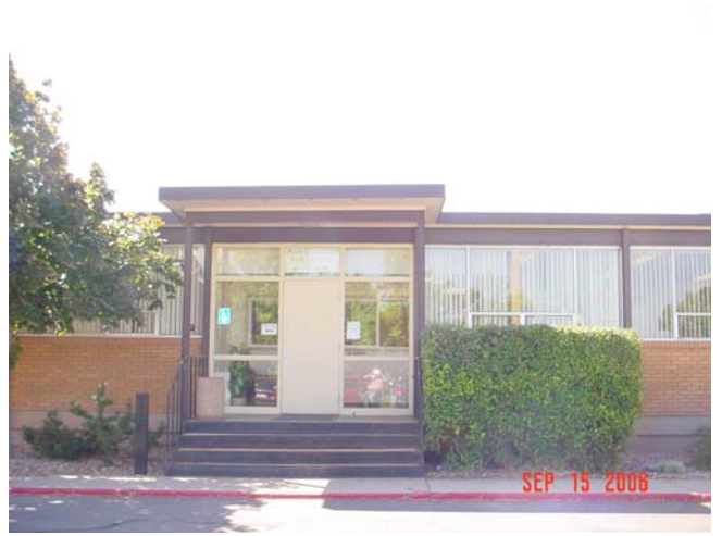
Photograph 8-SUU FACILTITES/AUTO View south, front entry to Facilities/Automotive building.
