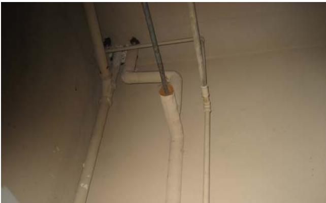
Photograph 5- T001 TSI Joints/Fittings, Mudded Room 111 Custodial No Asbestos Detected
