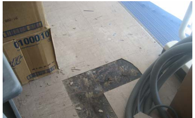
Photograph 6- M006 9" Floor Tile (mastic none detected) Level 500 Contains 10% Asbestos
