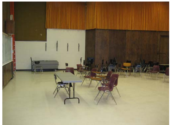
Photograph 12-SUU MUSIC BUILDING Room 209 (rehearsal), Asbestos Sheet Vinyl flooring (SVF-M004).
