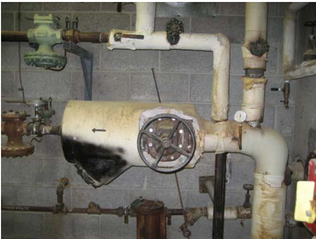
Photograph 15-SUU MUSIC BUILDING Room 111, Asbestos TSI valve body.
