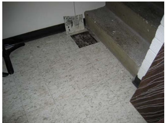
Photograph 10-SUU MUSIC BUILDING Room 100C stairwell, Asbestos 9" floor tile (M001).
