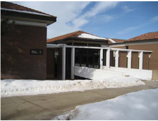
Photograph 1-SUU MUSIC BUILDING View northwest, front entry.
