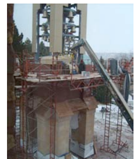
Carter Carillon Tower Under Construction
