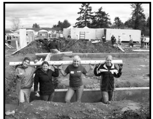
Students installing drainpipe for Habitat for Humanity alternative spring break
