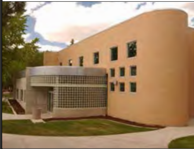
South Hall West Entrance
