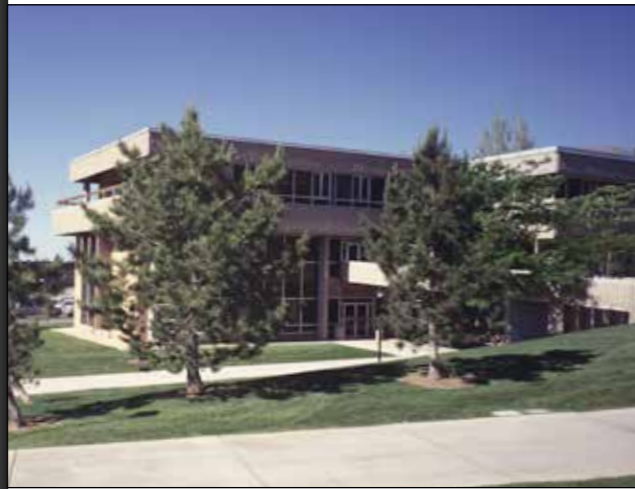
Bennion Administration Building
