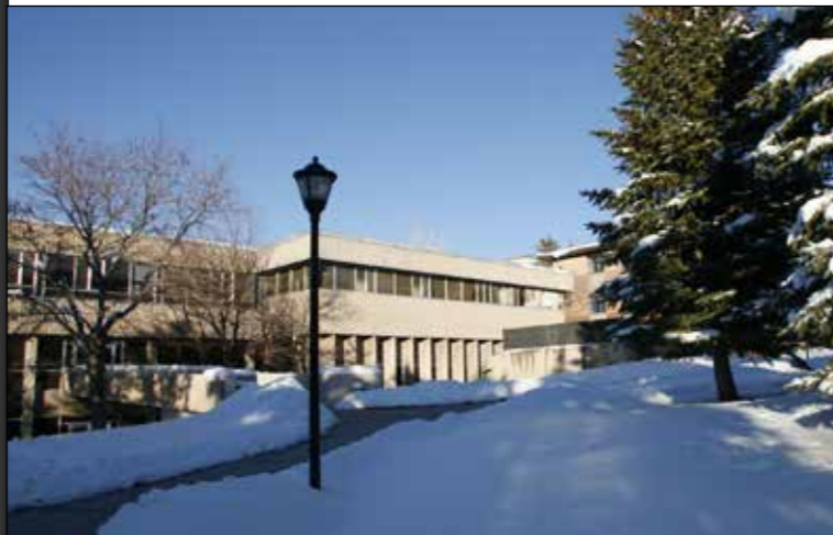
Bennion Administration Building
