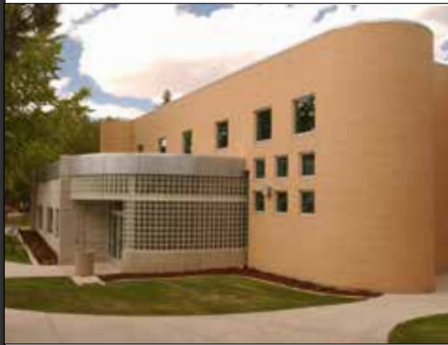
South Hall West Entrance
