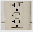
GFCI should be installed in any location with a potential water hazard.
